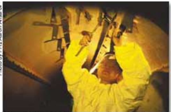
Petty Officer 3rd Class Thuy Bu, a Machinist's Mate on board USS McKee, removes the boiler internals.
