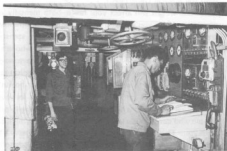
Standing watch in the fireroom at the Main Control Board are: BT2 D. W. Kashorek (left) and BT3 H. E. Robinson.
